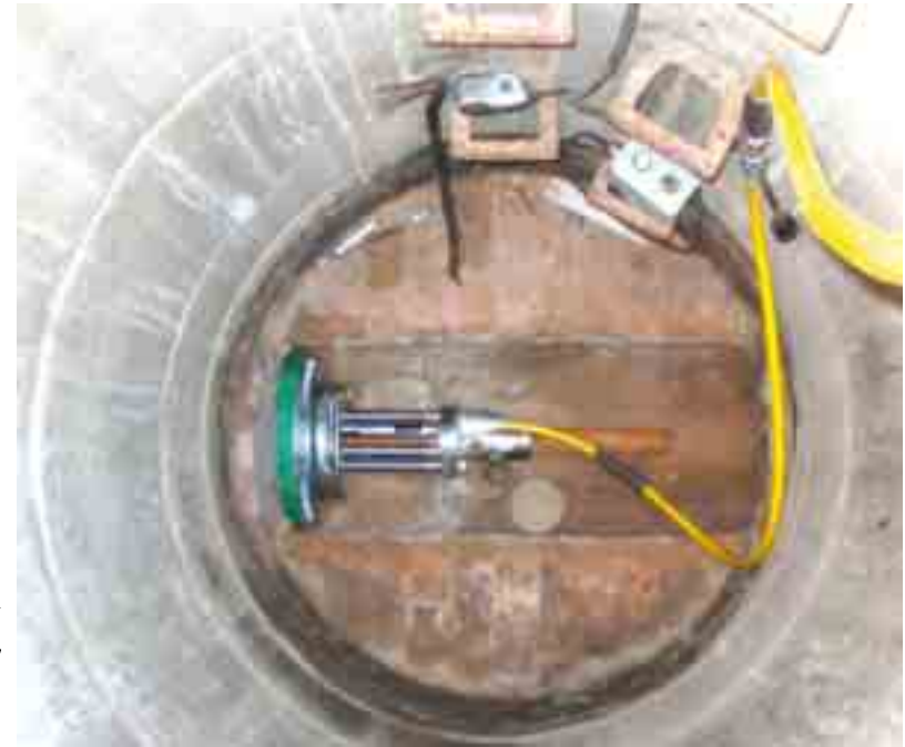
Guiding sleeve with gliding rollers (Patent pending)
