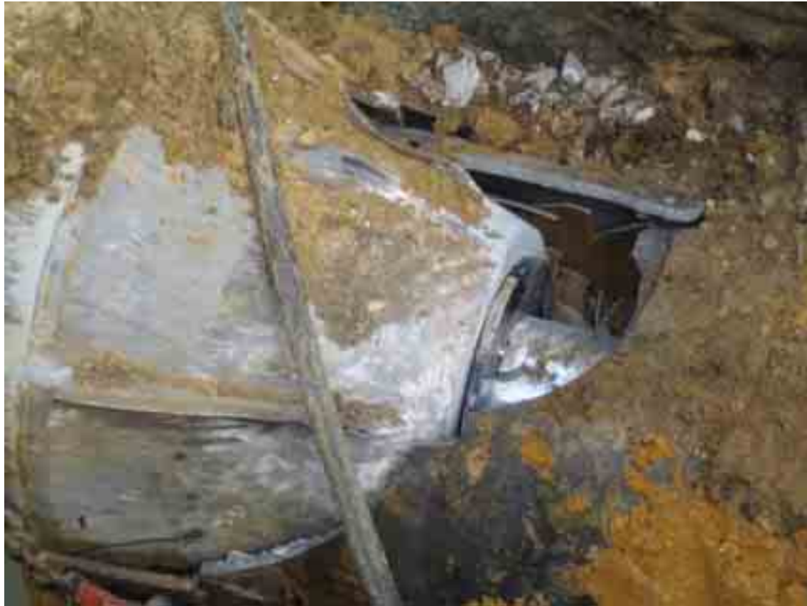
Bursting the old grey cast iron pipe ND 800
