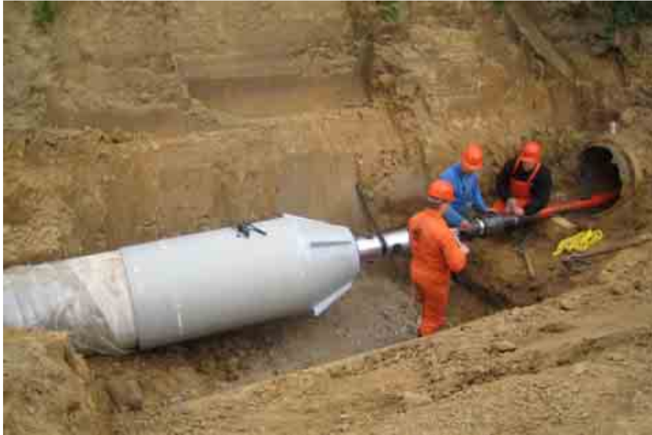
Preparation for pulling in the new steel pipe ND 800
