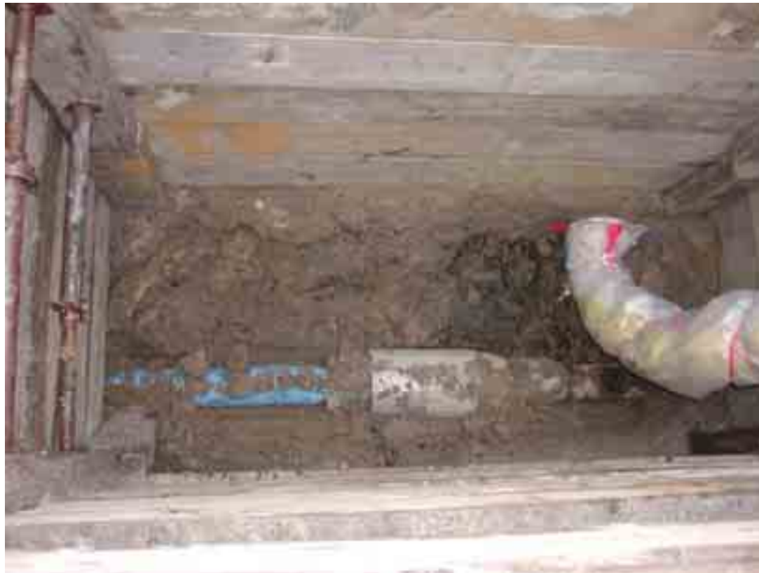
Pulling in the new cast iron pipe
