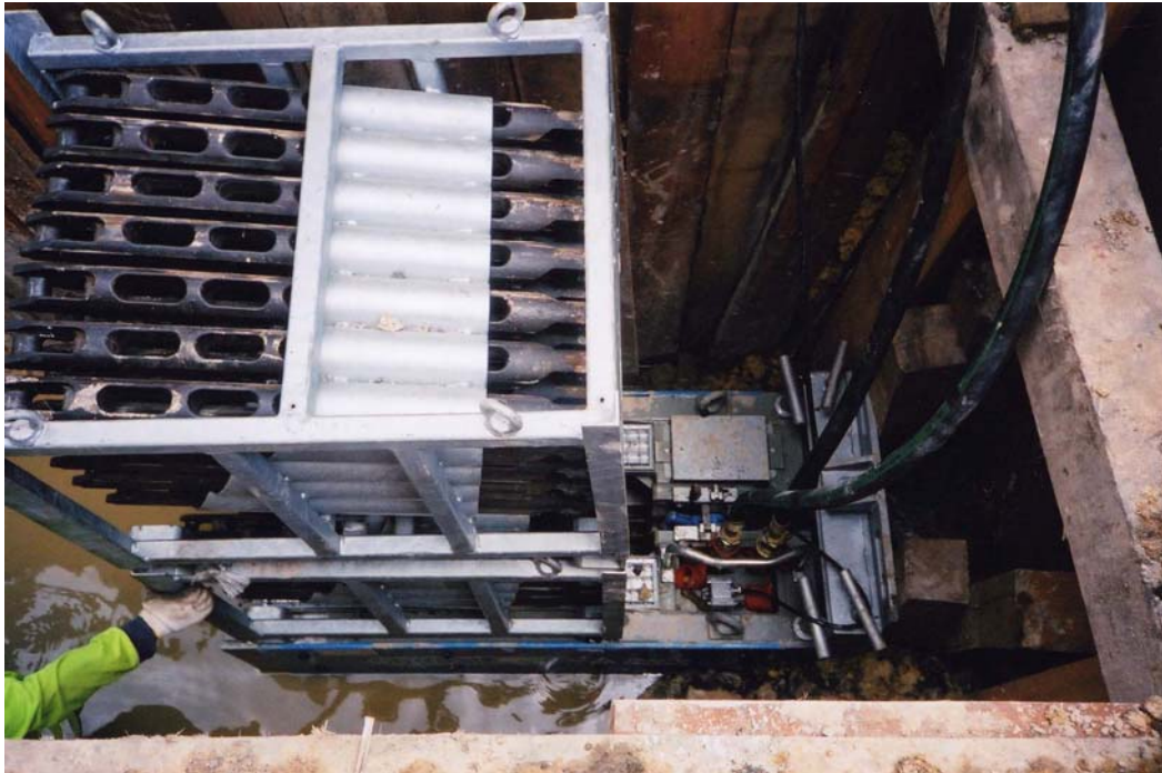
PHOTO 7: Note the unique rod storage boxes positioned on top of the GRUNDOBURST 800G. Each rod storage box houses 35 off 0.7 metre rods.
