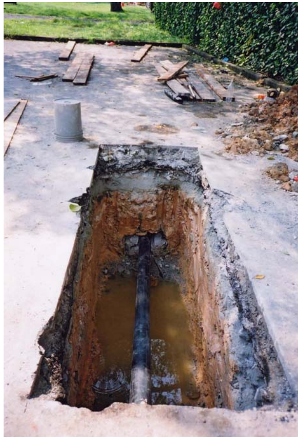
PHOTO 16 – View of 125mm PE pipe in the receive pit where a temporary connection to the existing sewer will be made until the next day's burst.
