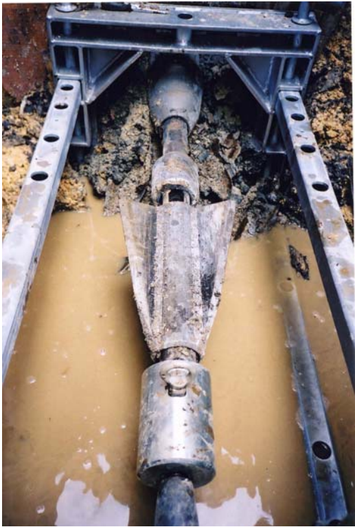
PHOTO 14 above – Shows the tooling arriving in the trench.
