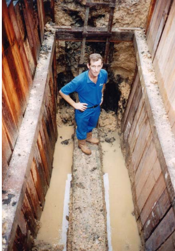
PHOTO 5 – In places the concrete measured 500mm x 500mm square.
