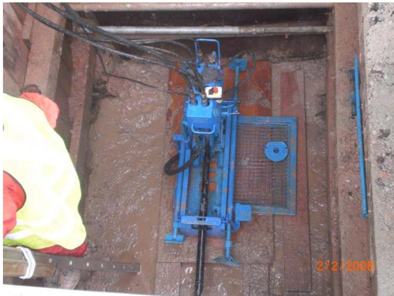
The entry/equipment pit was about 3 meters on width, 4 meters in length and 5 meters in depth. The reason to go so deep was to avoid the monsoon drain that was directly in front of the pit.
