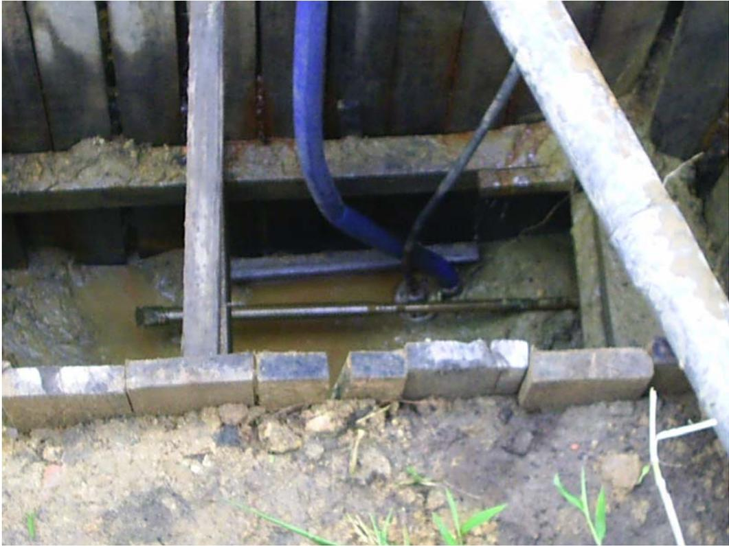
The drill head arriving on target at the exit pit. Total time taken was about 30mins.
