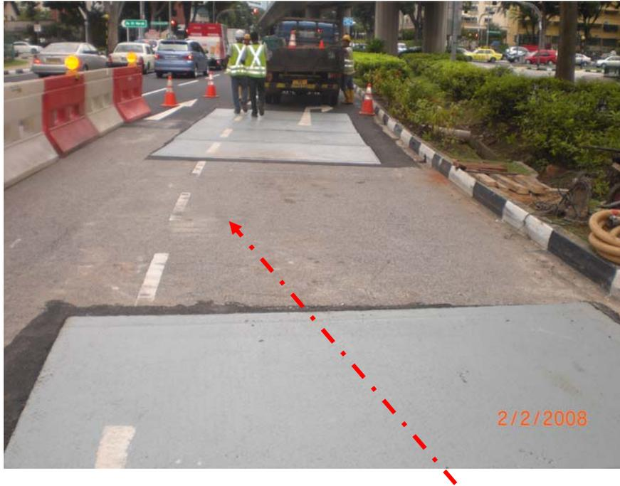
The objective of this job was to pull a Ø400mm HDPE pipe across the above drain culvert using trenchless method. Total length across the highway was about 14 meters.
